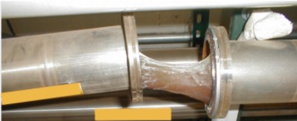
Figure 1- Chlorosilane polymer build-up in exhaust system from an epitaxial deposition system.
