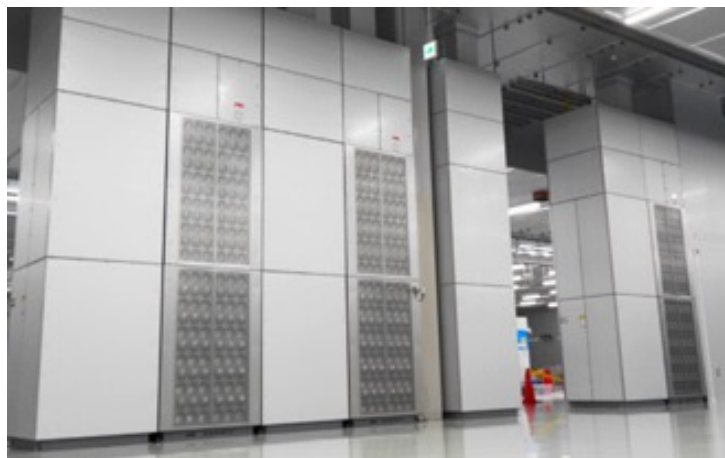
Figure 4- Swirling induction HVAC system (courtesy Fujitsu Semiconductor).
