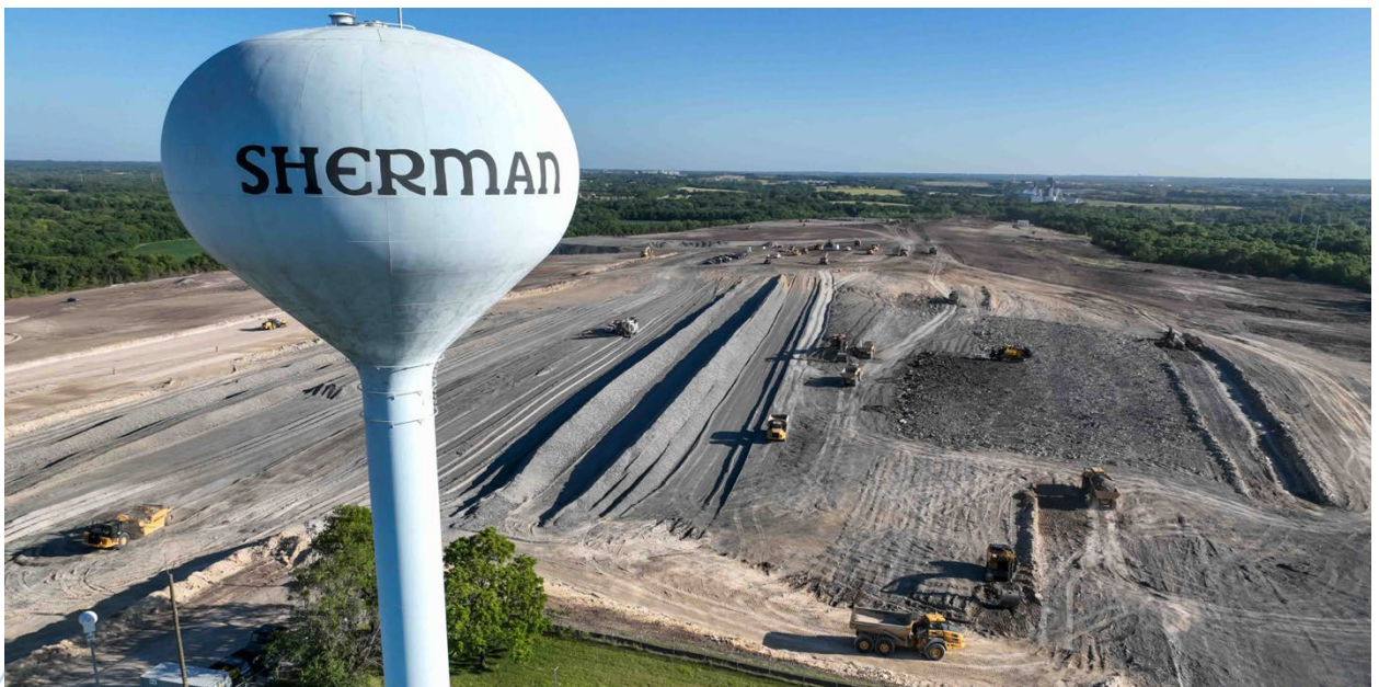
Figure 3- Texas Instruments Sherman fab complex during site preparation process.
