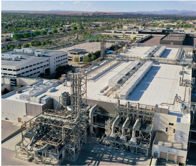
Figure 2- Example of a central utilities building attached to a wafer fabrication facility
