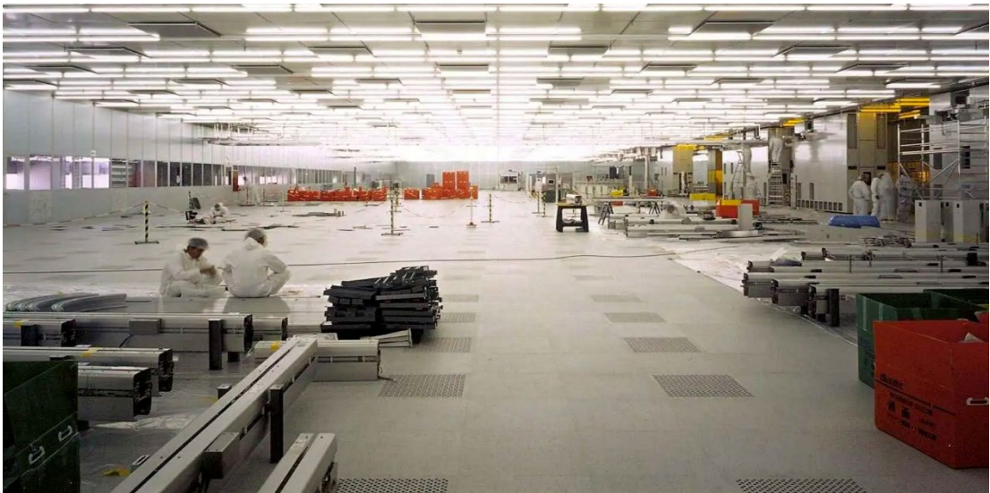
Figure 2- Picture showing a ballroom-style cleanroom nearing completion of construction
