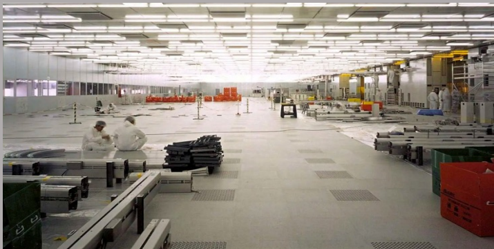
Figure 1- Picture showing a ballroom-style cleanroom nearing completion of construction.
